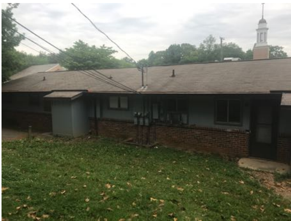
Photo 3 - Building 1 "C" side view
