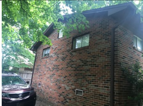
Photo 16 - Building 4 "D" side view
