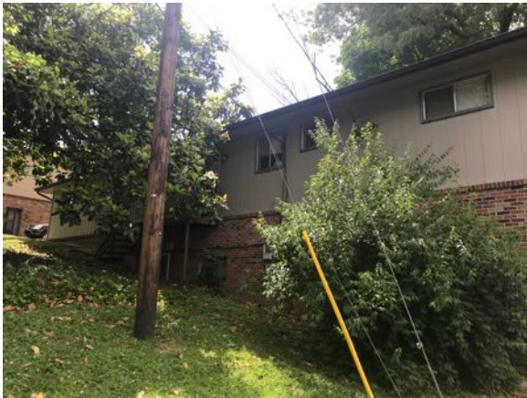
Photo 11 - Building 3 "C" side view
