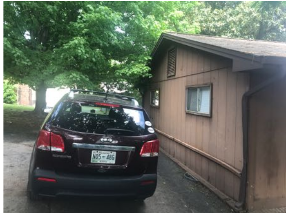
Photo 6 - Building 5 "B" side view
