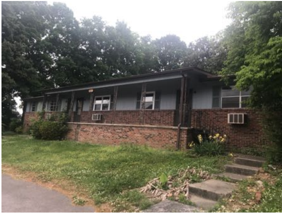
Photo 1 - Building 1 "A" side view
