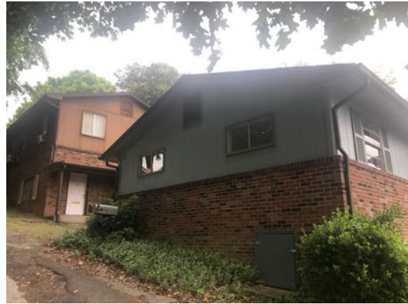
Photo 2 - Building 1 "B" side view
