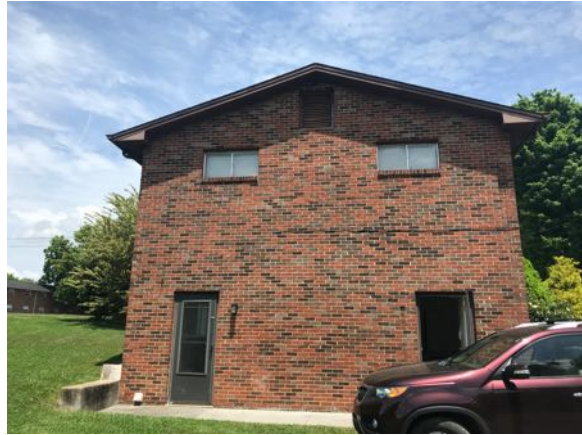
Photo 26 - Building 7 "B" side view
