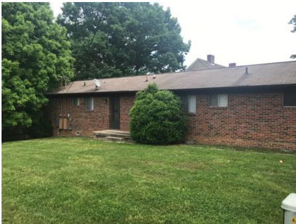
Photo 15 - Building 4 "C" side view
