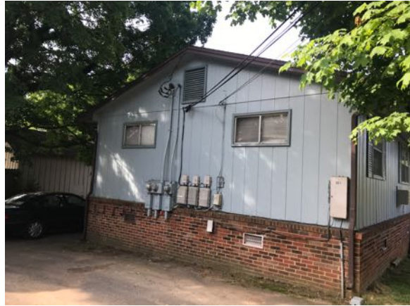
Photo 22 - Building 6 "B" side view
