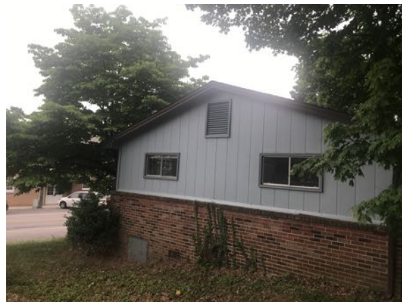
Photo 4 - Building 1 "D" side view
