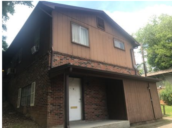
Photo 8 - Building 2 "D" side view
