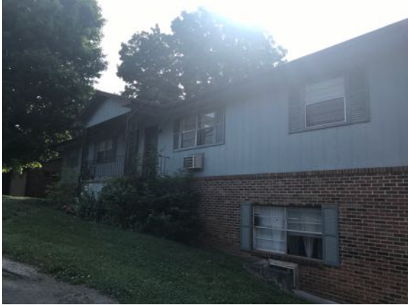
Photo 21 - Building 6 "A" side view
