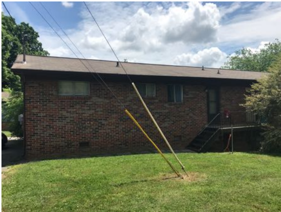
Photo 27 - Building 7 "C" side view
