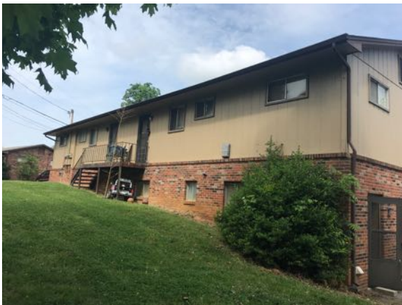
Photo 19 - Building 5 "C" side view
