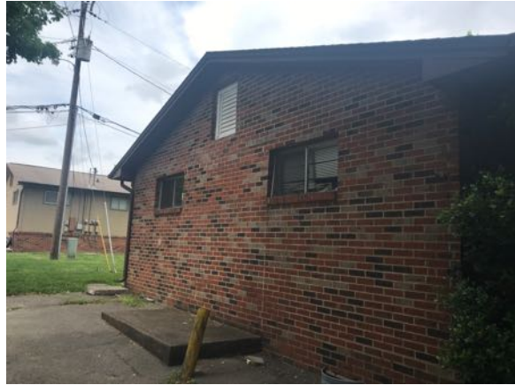
Photo 14 - Building 4 "B" side view
