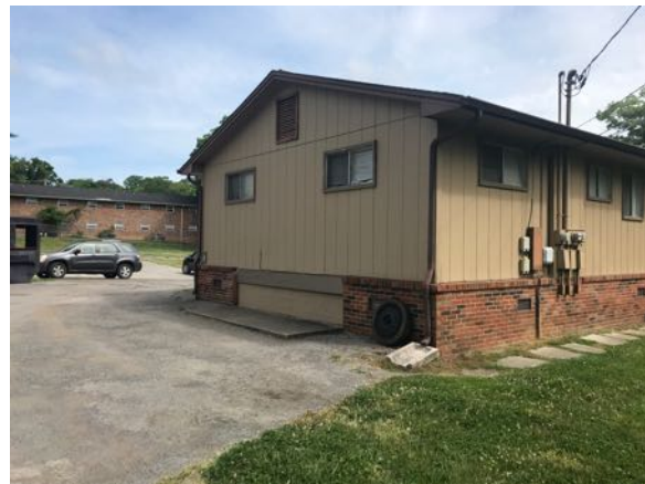
Photo 20 - Building 5 "D" side view
