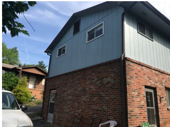
Photo 24 - Building 6 "D" side view
