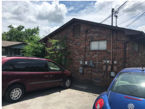
Photo 28 - Building 7 "D" side view
