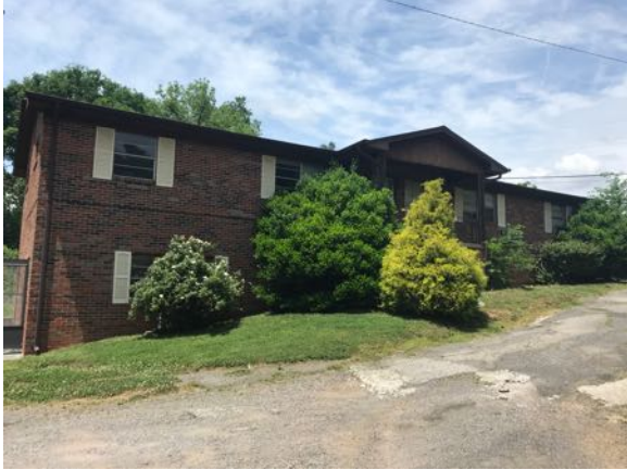
Photo 25 - Building 7 "A" side view
