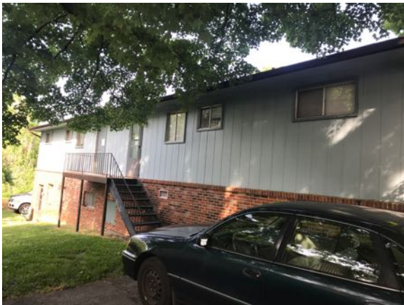
Photo 23 - Building 6 "C" side view
