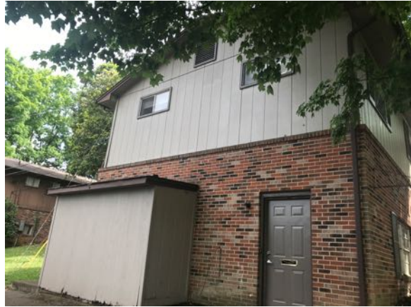
Photo 10 - Building 3 "B" side view
