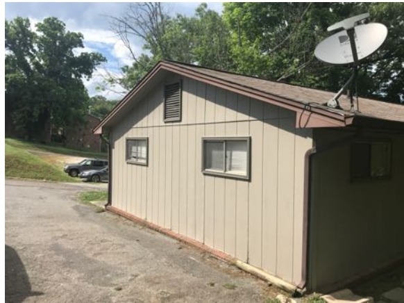
Photo 12 - Building 3 "D" side view
