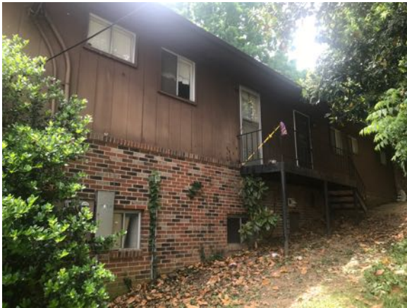
Photo 7 - Building 2 "C" side view
