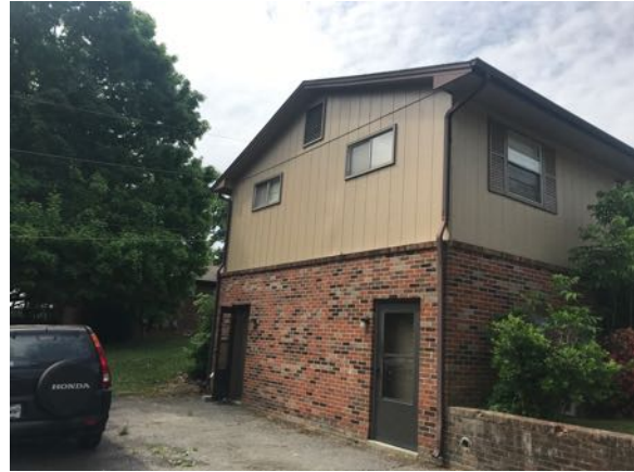
Photo 18 - Building 5 "B" side view
