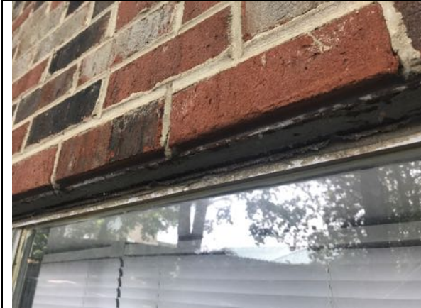
Photo 29 - Typical window/door lintle - POSITIVE
