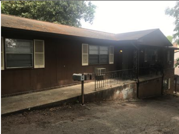
Photo 5 - Building 2 "A" side view
