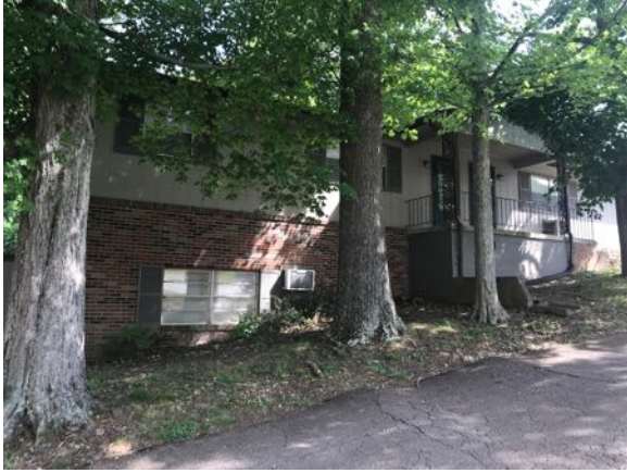
Photo 9 - Building 3 "A" side view
