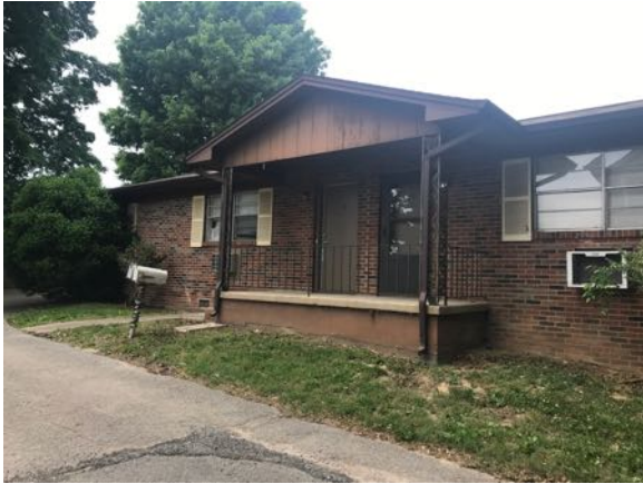
Photo 13 - Building 4 "A" side view
