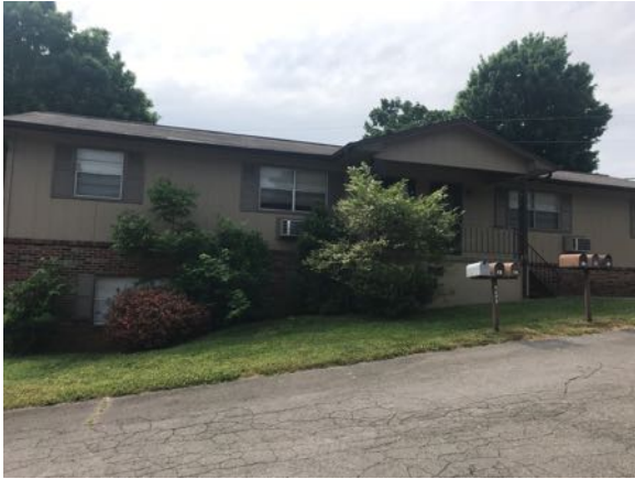
Photo 17 - Building 5 "A" side view
